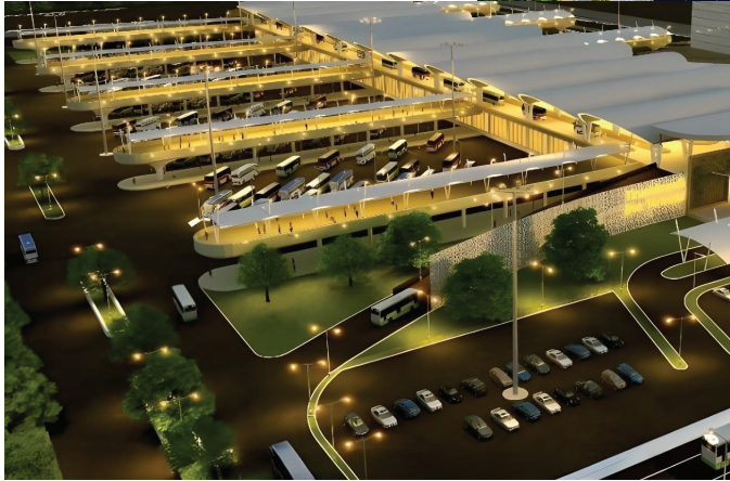
Panjapur Integrated Bus Terminus, Tiruchirappalli
